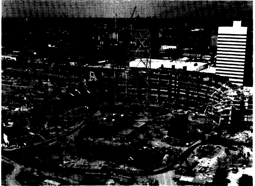
'Coliseum like' SkyDome takes shape. ▶
