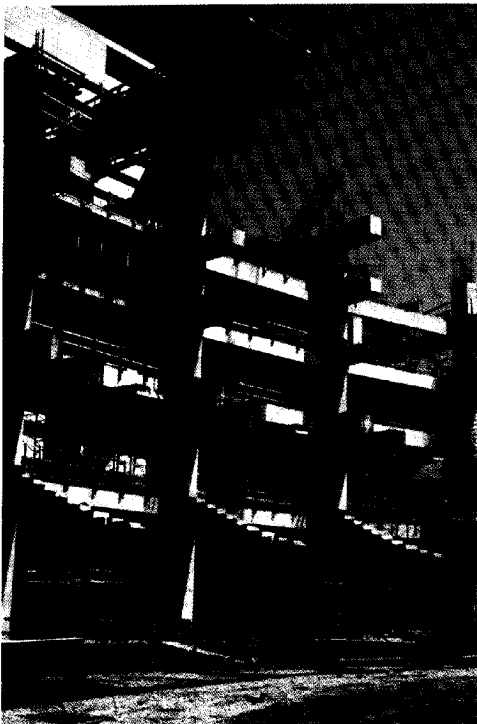
◀ Cantilevered beams provided unobstructed views.
