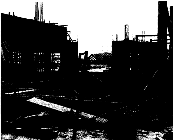
Simultaneous erection of portions of two floors allowed early starts for other trades.
