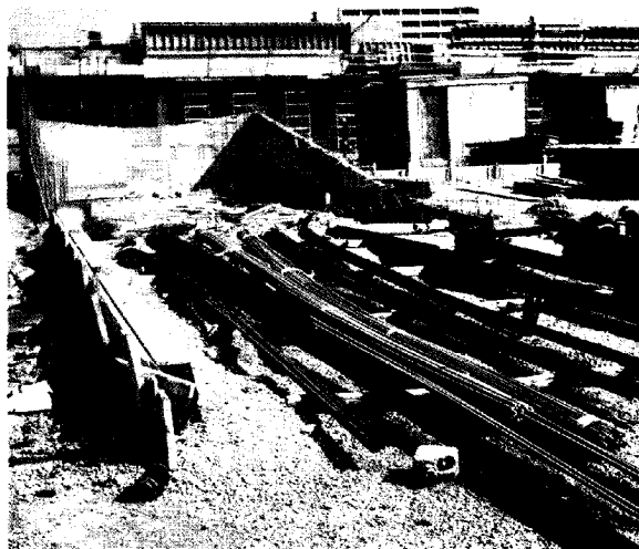
▲ Reinforcement, formwork and concrete had to be "hop-scotched" around the site.
